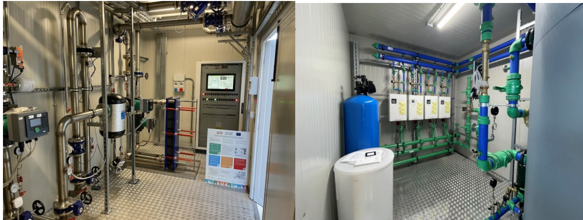
Figure 3: construction works (Ospitaletto).
